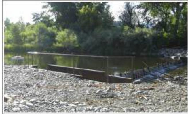
**Figure 21 Before:** A gravel and wood “push-up” dam that blocks fish passage on the upper mainstem John Day River, south of John Day... **And after!** The lay-flat stanchion dam includes a channel for fish to migrate past the dam. When the dam is lowered, the stream flows naturally (photos and caption from BPA 2009).
