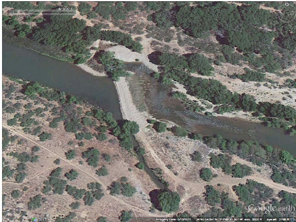
Figure 6.12. Aerial view of the Hickey ditch diversion dam. See fig. 6.11 for location. North is at top. Verde River flows around north end of the diversion dam and returns immediately to its natural channel. The diverted portion of the Verde River is visible flowing southeast in the bottom-center part of the image. Google Earth Imagery date 6/13/2011.
