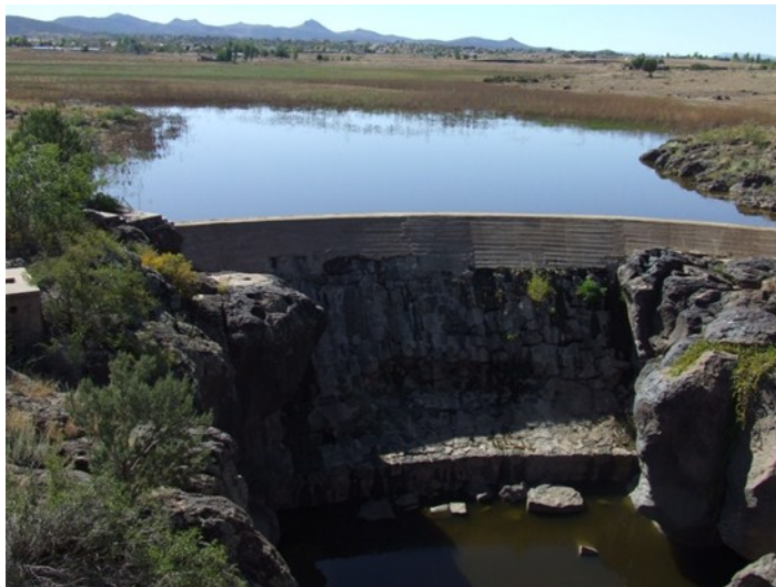
Figure 3. Low concrete dam that forms ephemeral Sullivan Lake. Dam, about 115 feet wide, is set into the head of a narrow steep-walled canyon cut into basalt. The dam marks river-mile zero on the Verde River, although continuous perennial flow now begins about two miles below the dam. View is westward.
