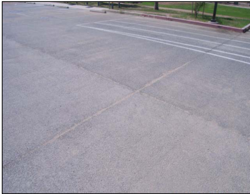
Photo 5.4 Pervious Concrete Installation
