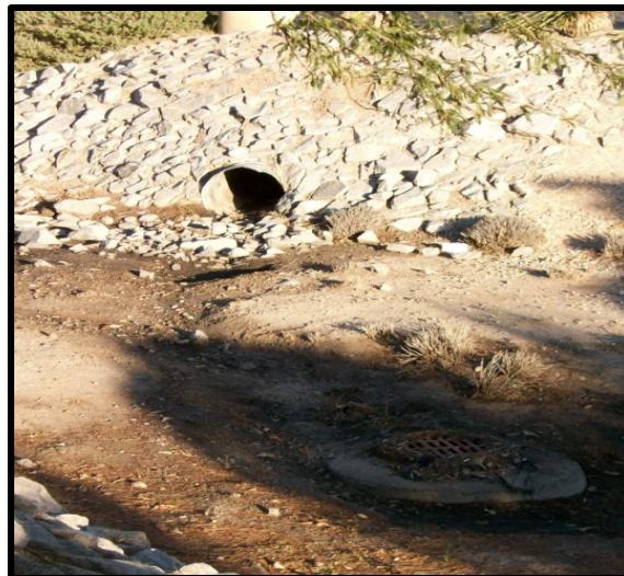
Photo 4.5 Detention Basin Dry Well Installation
