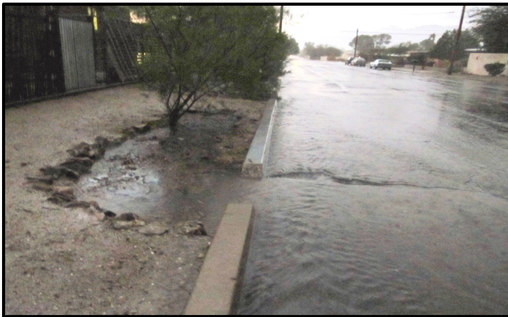
Photo 2.1 Roadside Stormwater Harvesting Basin at Full Depth
