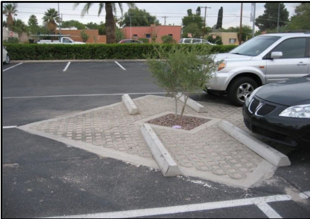
Photo 5.2 Concrete Grid Pavement Installation
