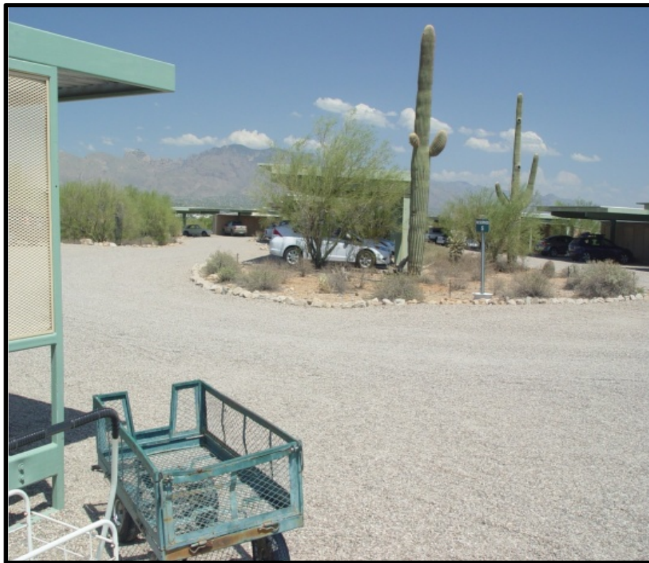
Photo 5.1 Porous Gravel Installation
