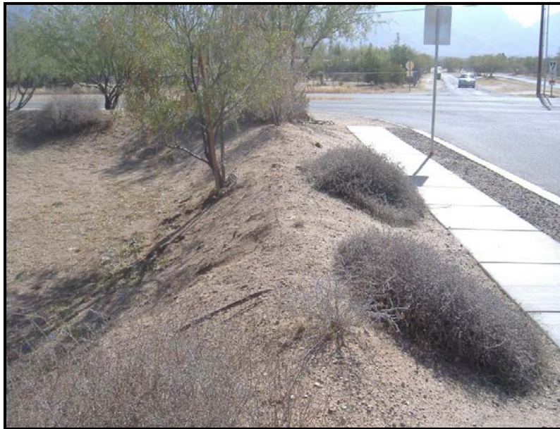
Photo 4.4 Residential Subdivision Basin with Embankment
