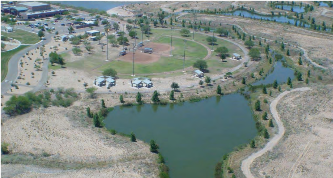
Stormwater and reclaimed water are used in the Kino Environmental Restoration Project
