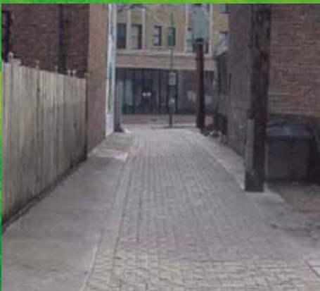
Chicago alley retrofitted with permeable pavement
