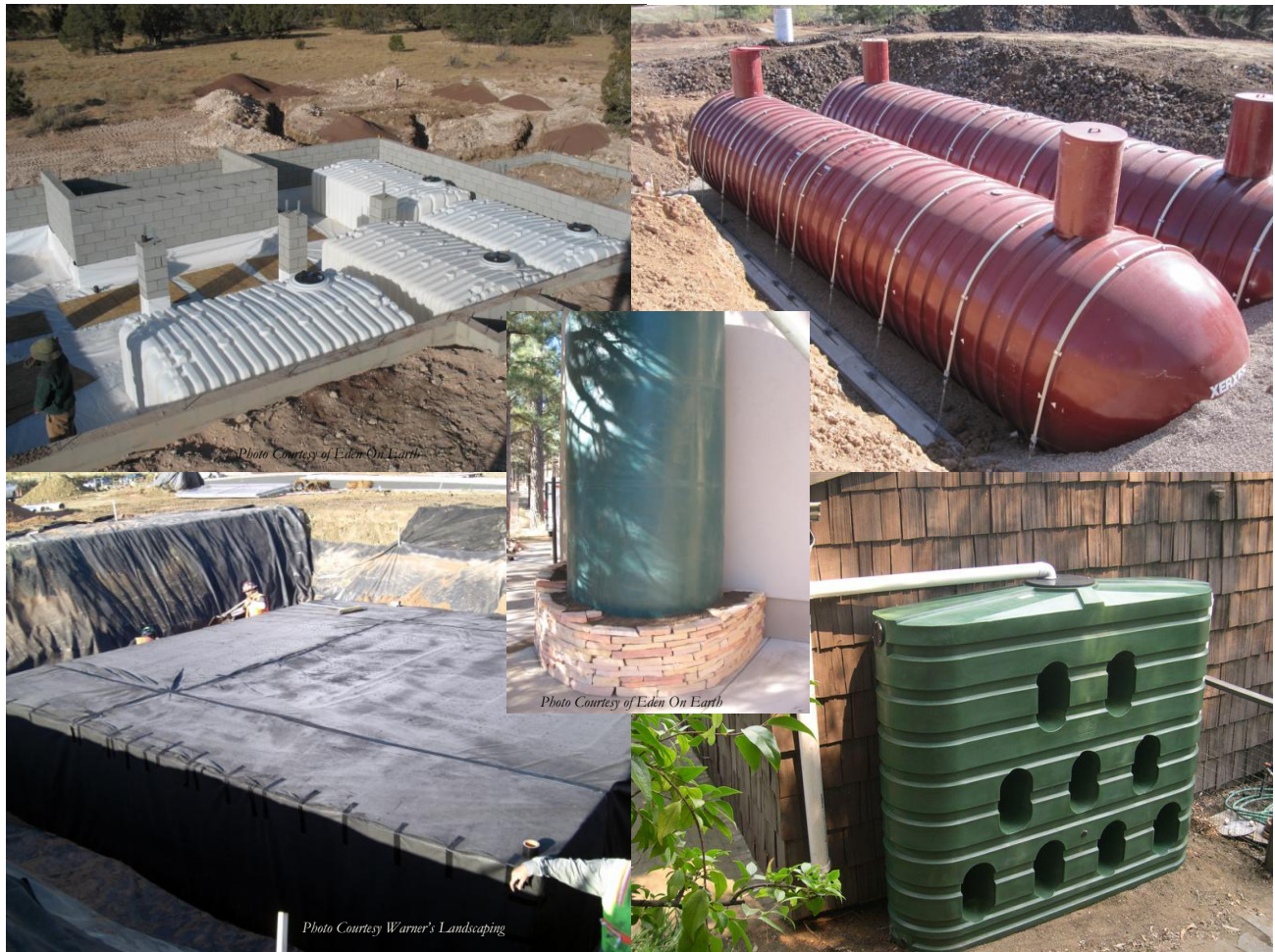
Figure 6.1- Various types of rainwater storage tanks. Clockwise from top left: Rainwater storage in a crawlspace, underground fiberglass cisterns, Bushman® tank, modular and stackable underground cistern, and aboveground cistern with knee wall (center).
